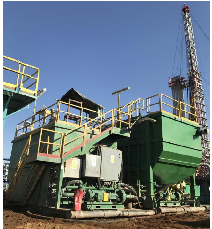
Fig. 01 – High-Volume Dewatering System.
