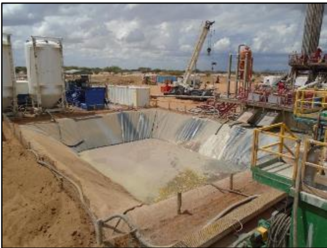
Fig. 03 – Remaining Waste Pit volume at High-Volume Dewatering System Rig Down. (Well #5)
